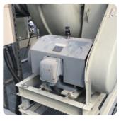
MOCOM-VT monitors the physical aspect through its wireless vibration and temperature sensors. The edge computing capability of MOCOM-VT empowers it analyze the abnormal vibration through harmonic frequency and component. For temperature detection, it detects not only the motor temperature, and also performs simultaneous comparison with temperature sensor on wireless gateway (MOCOM-DC) to avoid false alarm due to environmental factors.
